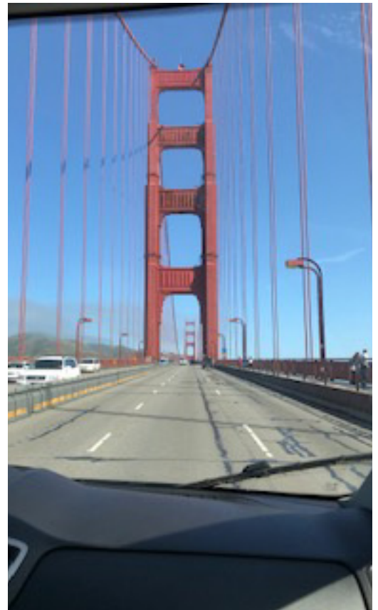
Golden Gate Bridge, San Francisco, CA 2020
